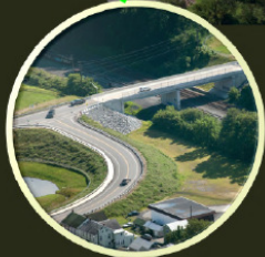
Railroad Bridge and Access Ramp
