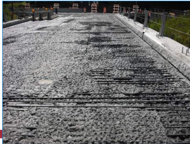
Post-Hydrodemolition
